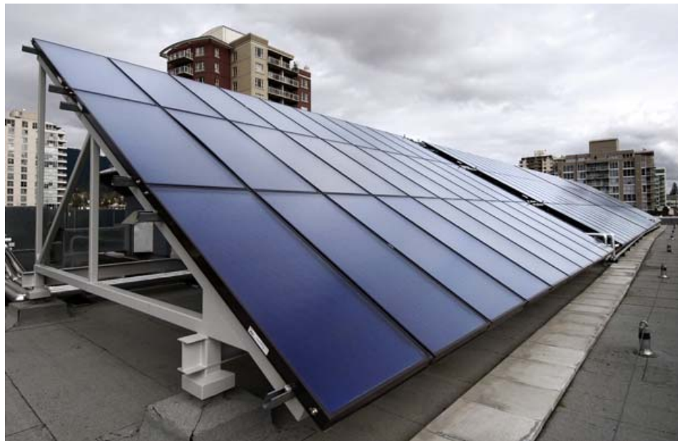
Figure 21 - Solar Hot Water Panels - North Vancouver
