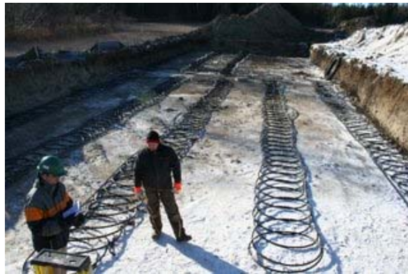
Figure 15 - Installing a Ground Source Heat Pump Field
